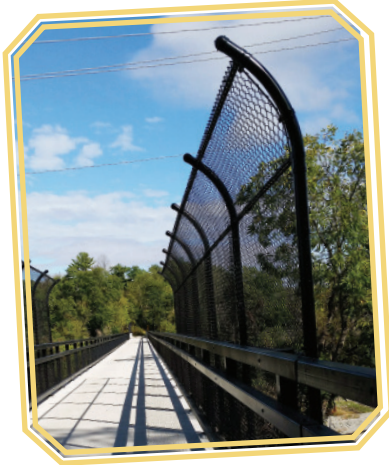
The new Library Viaduct Bridge sits at Mile 35.6.
