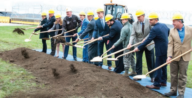
Col. Jeffrey Van Dootingh (fourth from left), commander of the 911th Airlift Wing, is joined by Lt. Gov. Mike Stack (fifth from left), construction company representatives, local officials, and representatives for state officials for a groundbreaking at the Air Force Reserve base Nov. 7.
