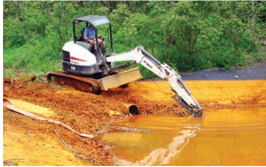
ABOVE: An excavator stirs medium in an impoundment on a pond managed by the Montour Run Watershed Association. Iron oxide is responsible for the orange coloration. BELOW: Montour Run is considered impaired by the state but has been improving. PHOTOS SUBMITTED
